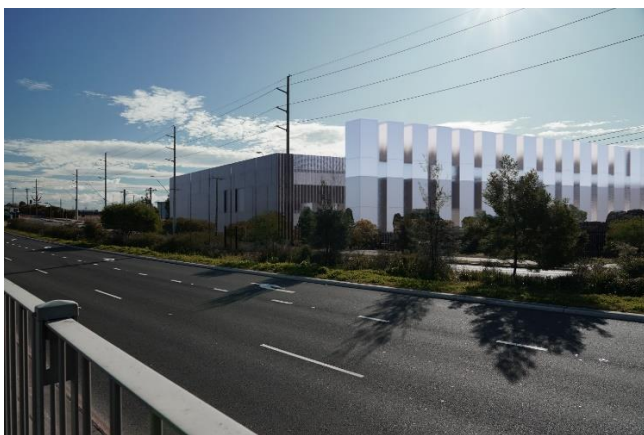
From Old Wallgrove Road facing West
