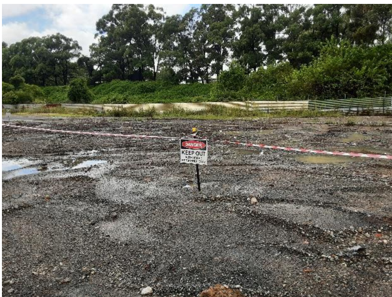
Photo 13 Disturbances throughout the study area, with large portion of site cordoned off due to asbestos, facing south-east
