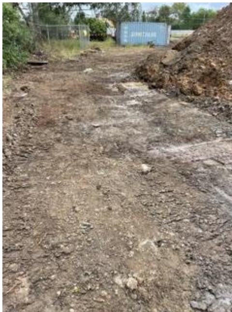
Photograph 3 – Removal area subsequent to remediation works
