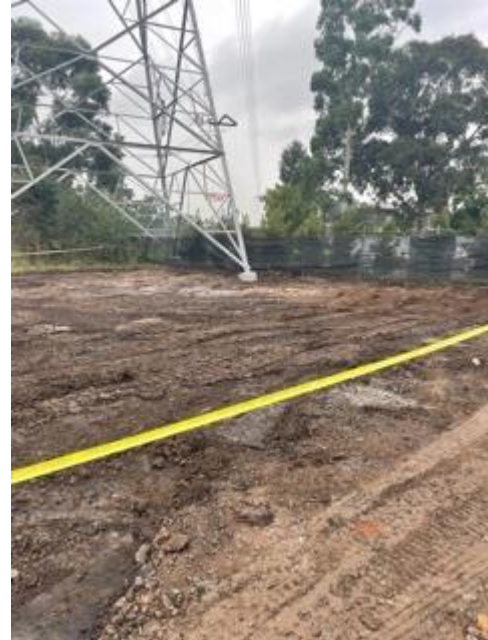
Photograph 2 – Removal area subsequent to remediation works
