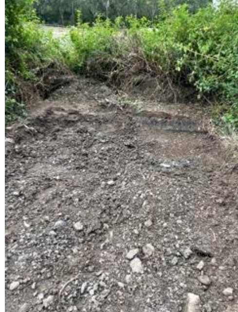
Photograph 2 – Removal area subsequent to remediation works
