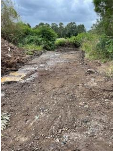
Photograph 1 – Removal area subsequent to remediation works
