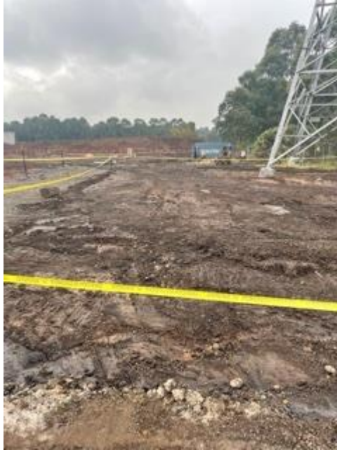
Photograph 1 – Removal area subsequent to remediation works
