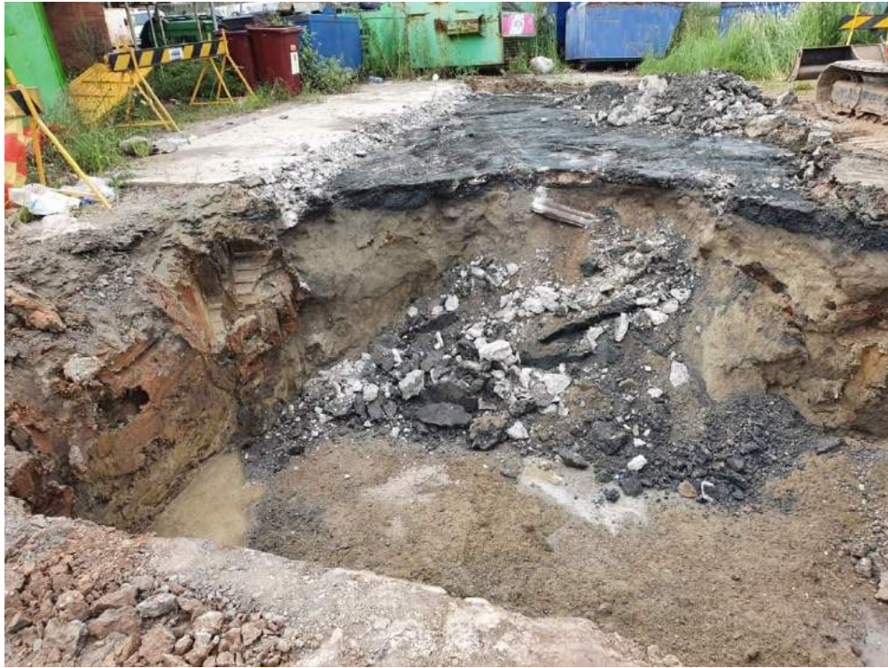
PHOTOGRAPH 3 Concrete and asphalt layer above Tank 3, looking east.
