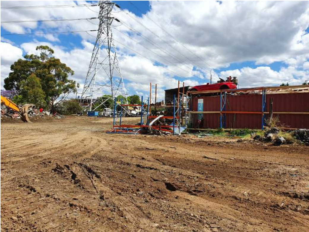
PHOTOGRAPH 7 Car wreckers portion, north west corner, view south east.
