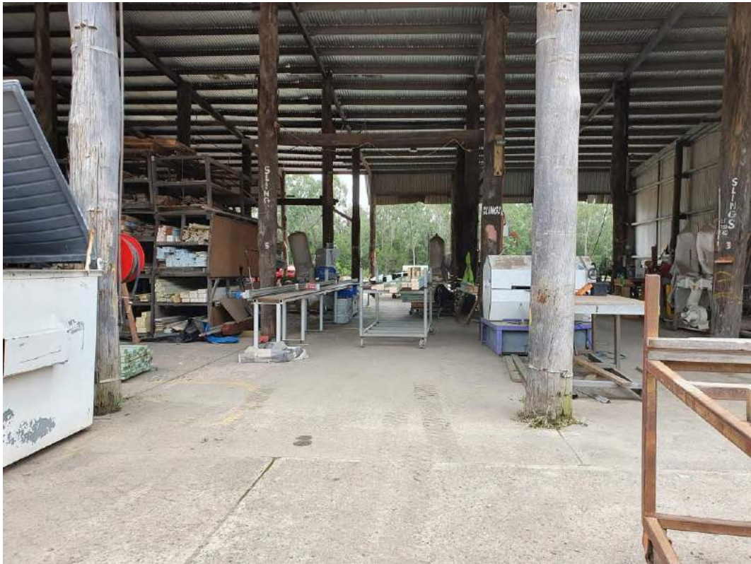
PHOTOGRAPH 1 Northern portion of the site view north through open building.
