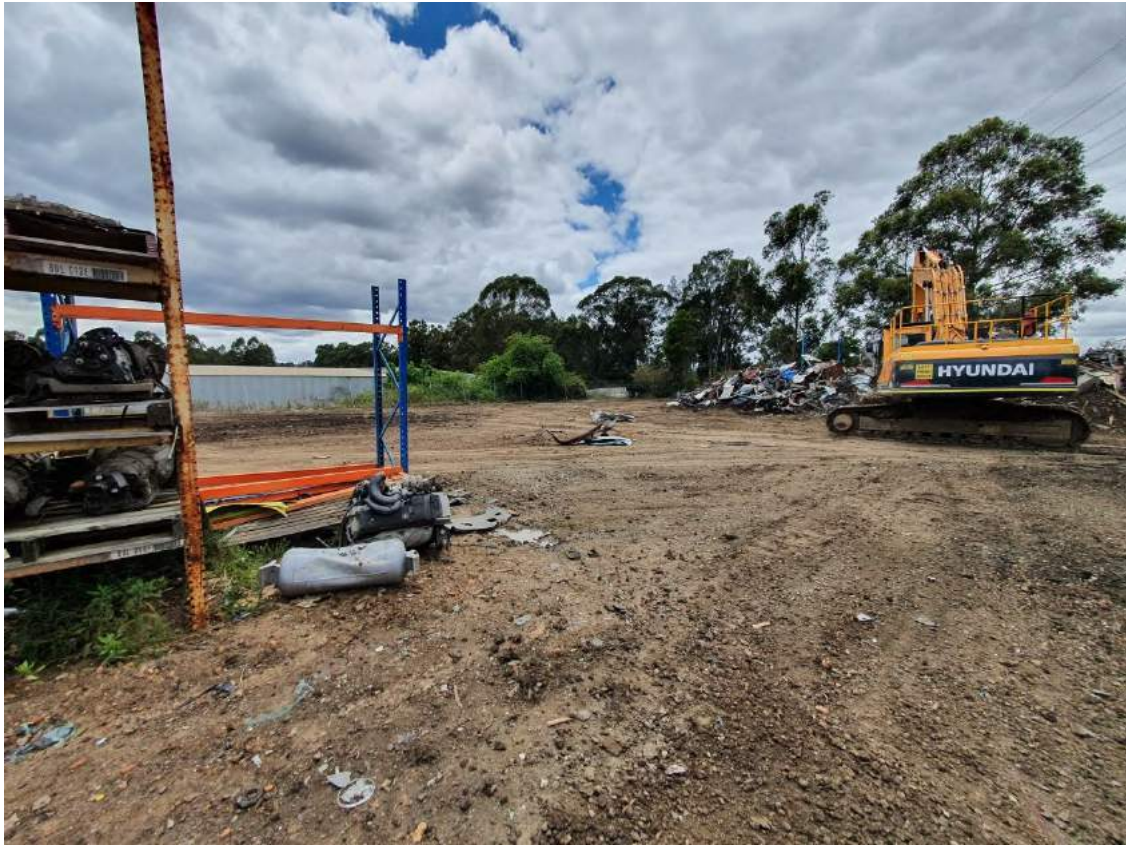
PHOTOGRAPH 5 Car wreckers portion, view north east from near S15.
