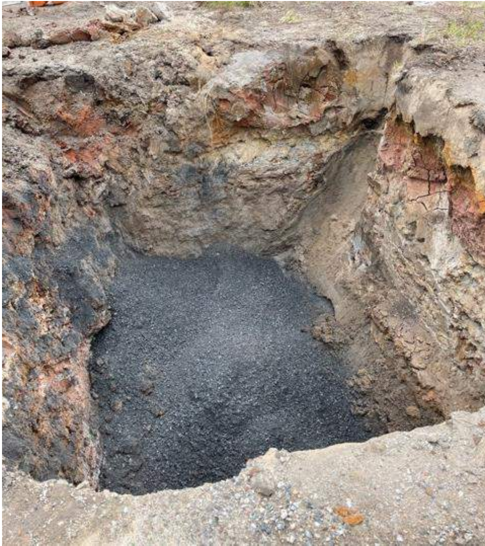
PHOTOGRAPH 10 Placement of clean backfill material within pit excavation by AIS.
