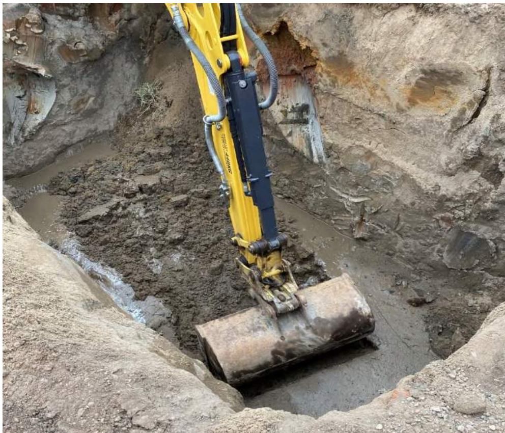
PHOTOGRAPH 4 Excavation of backfill sand material at base of Tank 2 pit.
