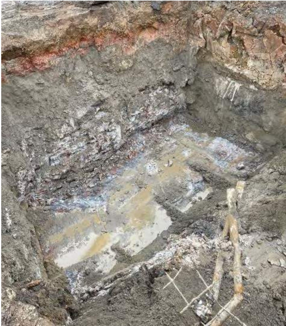
PHOTOGRAPH 9 Removal of backfill sand material by AIS from beneath Tank 2.
