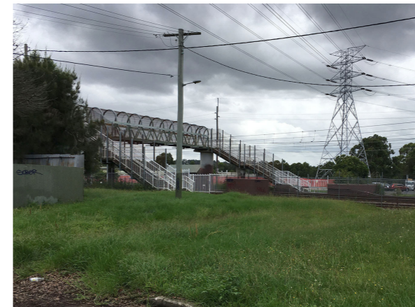
29 View towards the site from the McCoy Street turning circle on the western side of the railway line.
