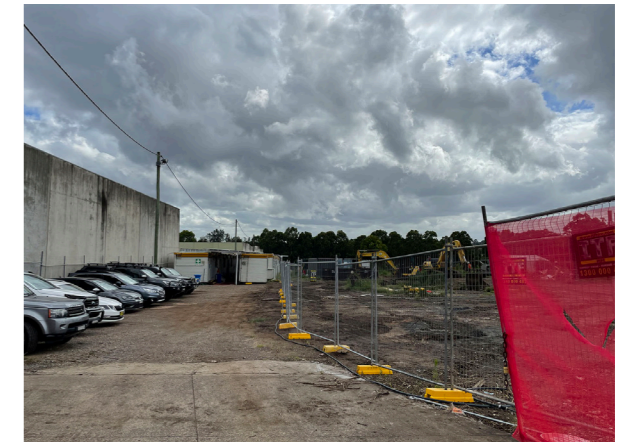
3 Access roadway off Station Road providing a connection to the south-west corner of the site.
