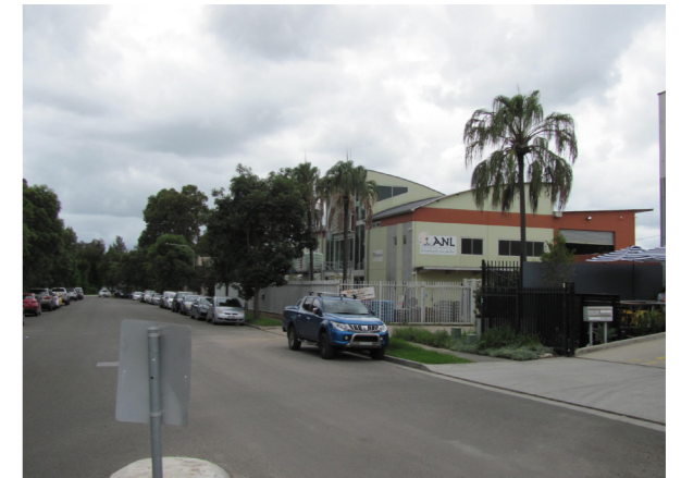
30 View north-east along Tollis Place.
