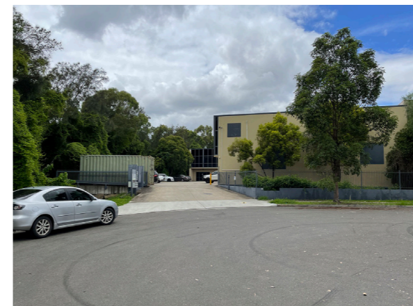
32 Commercial buildings located west of the site at 12 Tollis Place.
