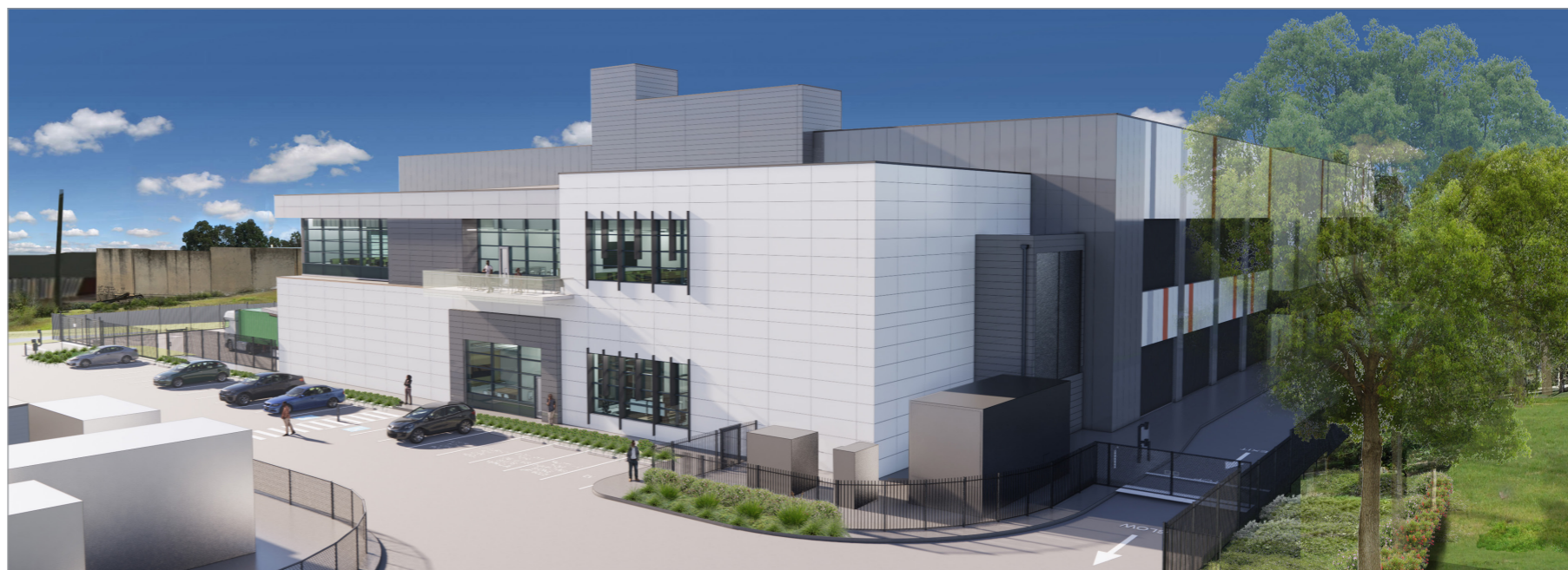
VIEW OF DATA HALL & ADMINISTRATION BUILDING FROM SOUTH
