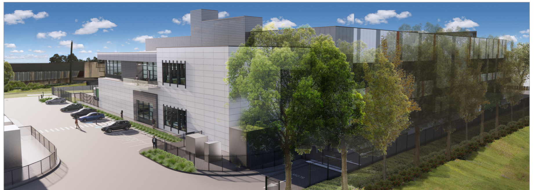
VIEW OF DATA HALL BUILDING FROM SOUTH
