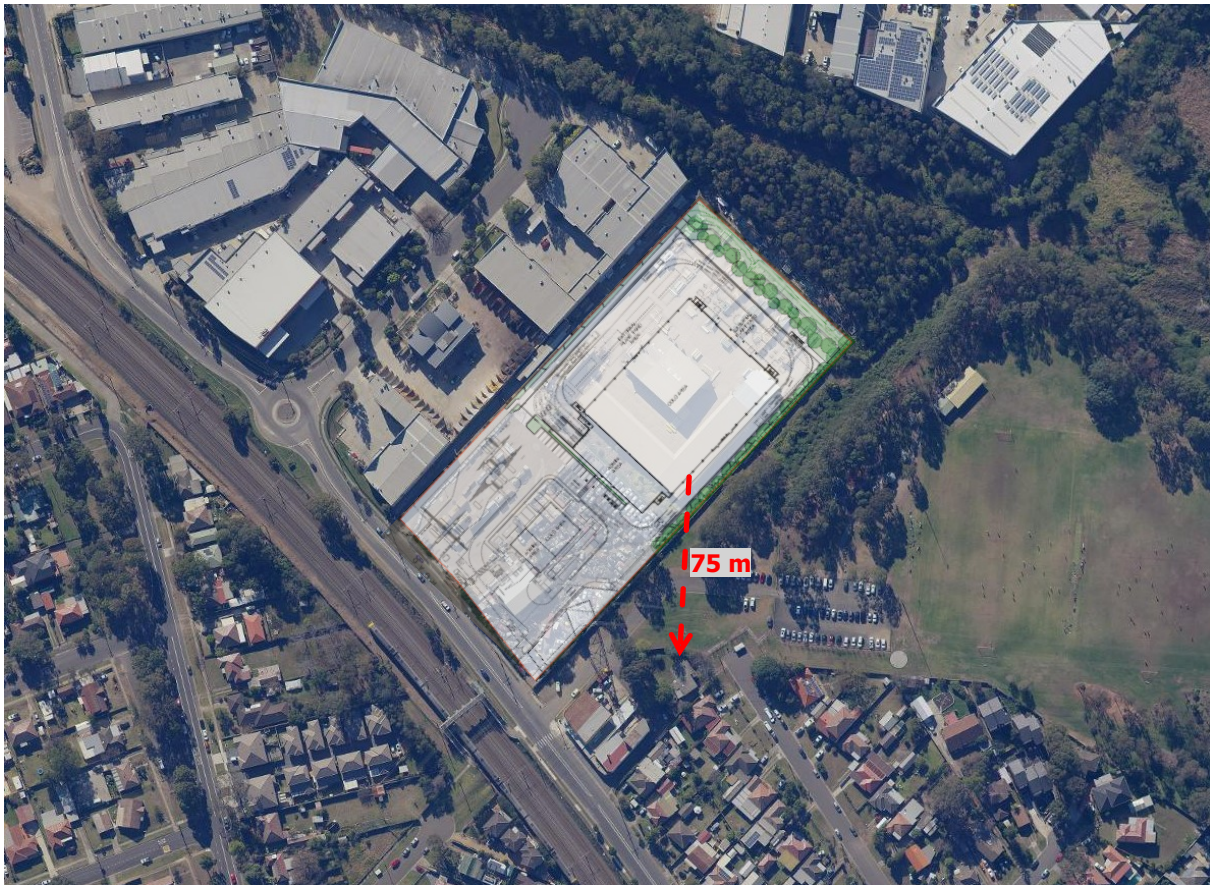
Figure 6 Proposed SYD08 datacentre location with respect to nearest residential receivers
