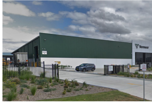
EASTERN CREEK DRIVE: CORRUGATED STEEL WAREHOUSE
